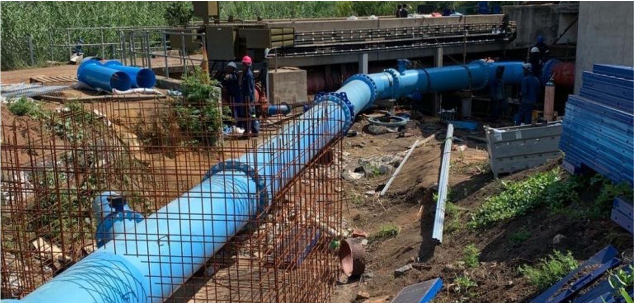
PIPELINE AND INFRASTRUCTURE FIELD EXPOSURE
